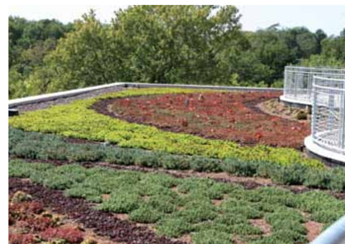
Green roofs create visual interest and save the energy.
