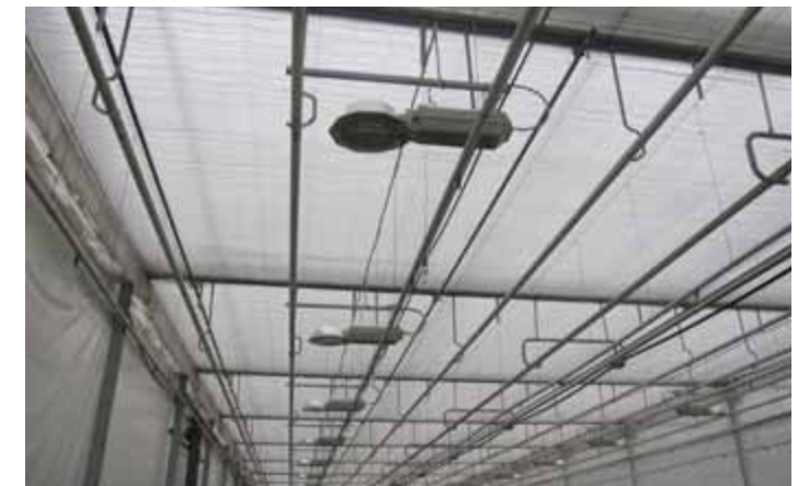
Close-up to show the energy screen, the HID lamps, and the mist line.
